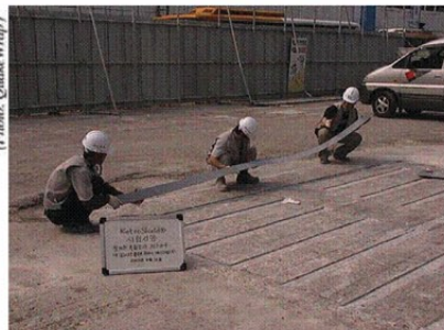
Figure 1: Installation of laminated carbon strips for strengthening a bridge deck.
